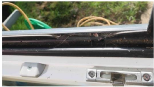
FIGURE 7 (right) one of two folds in the draught seal of the window to the left of the back door
