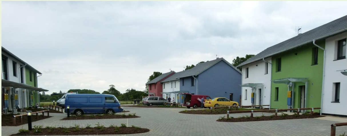
Figure 1: General View looking East: Houses to right, flats to left
