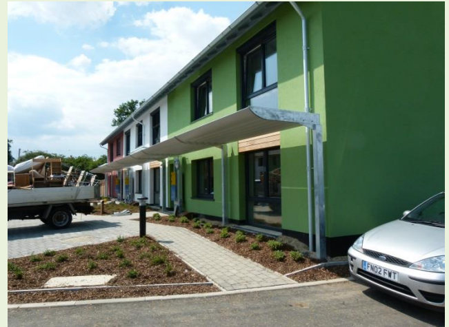
Figure 13: Flats with Brise Soleil (solar shading)
