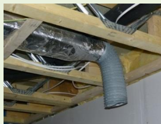
Figure 20: Joists and supply duct
