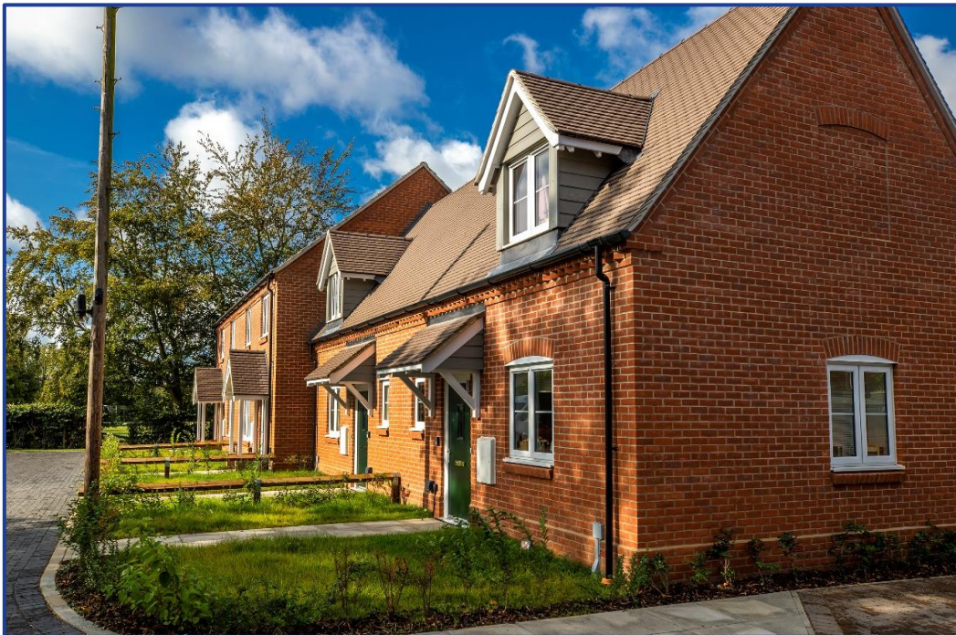
8 new homes completed in August 2023 at Stoke by Nayland, Suffolk
